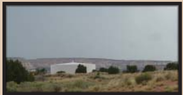
Acoma Well Site
