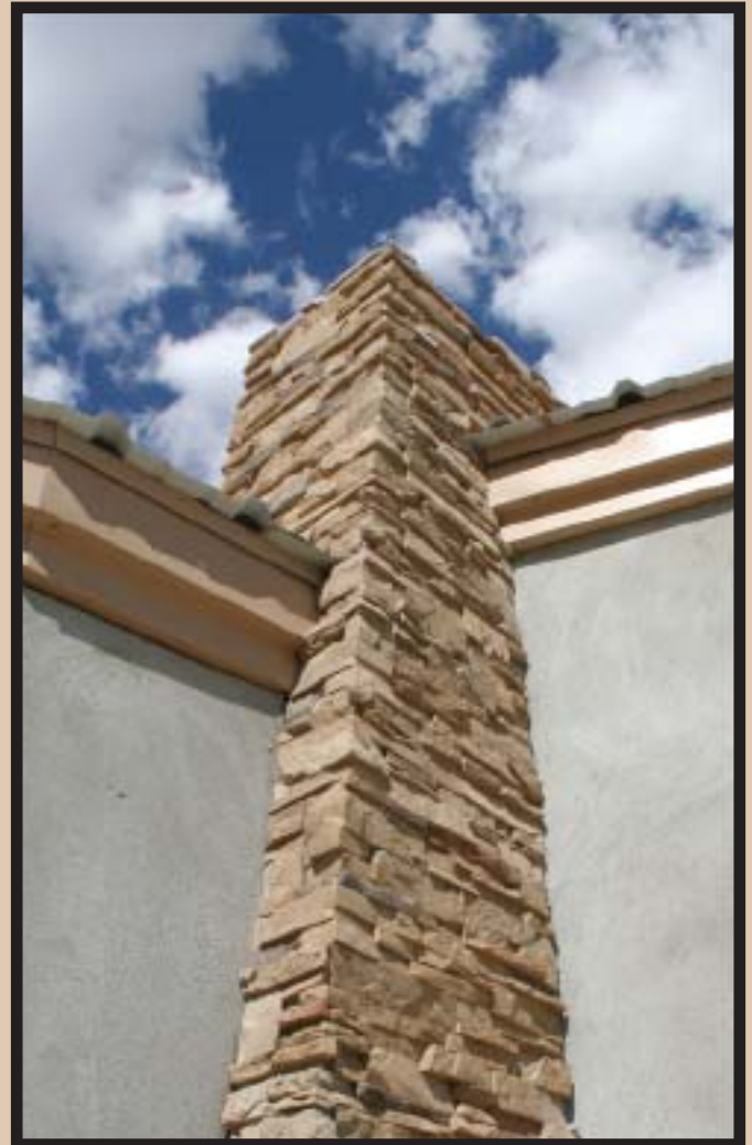
Smith Lake Veterans Center Project
