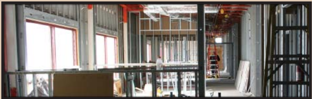
Smith Lake Veterans Center Project
